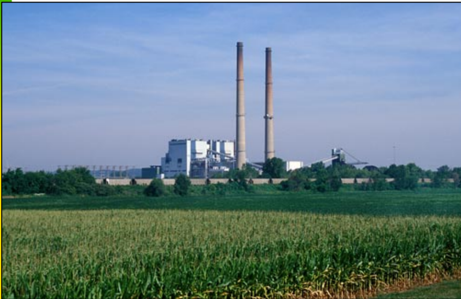
Portage des Sioux power plant near confluence of Missouri and Mississippi Rivers
